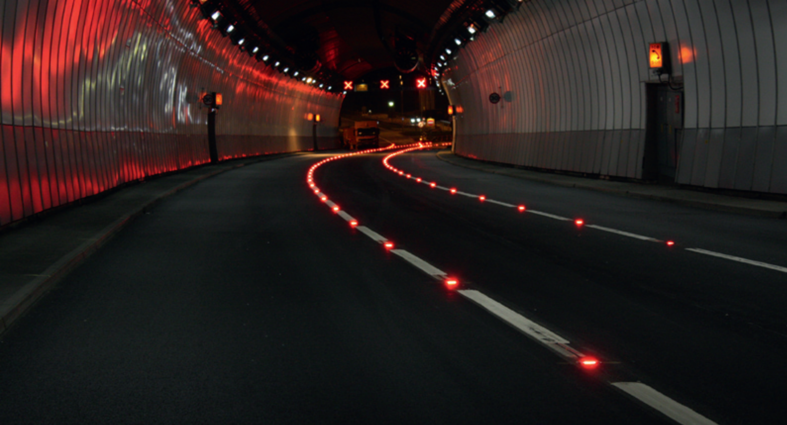
Saltash Tunnel, Cornwall, United Kingdom
